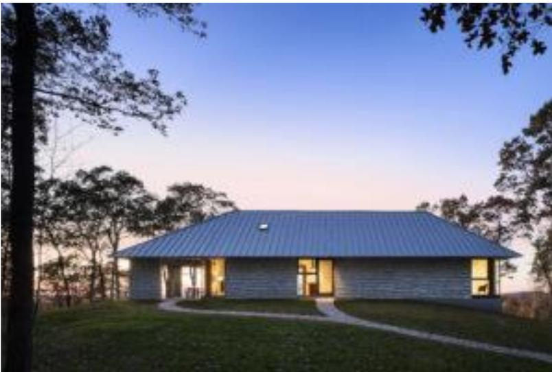
The exterior is clad in a natural handmade brick providing texture and thermal mass. Contrasting the cool appearance of the brick, window frames constructed of solid wood increase the R value of the glazing assembly.
