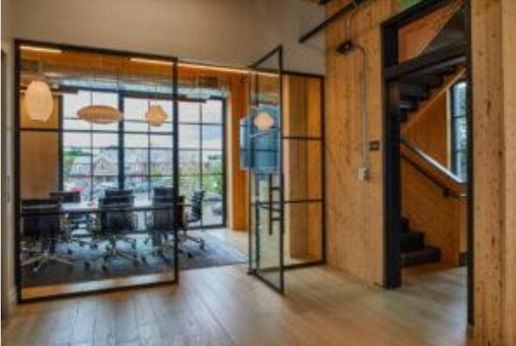
The project is among the first mass timber buildings in Connecticut using cross laminated timber as it's structural, walls, floors and ceiling systems. The use cross laminated timber as a finish material adds both warmth and coolness to the space. A fiber cement exterior skin applied over a rain screen provides a crisp and environmentally friendly exterior expression. A roof deck expands the office environment to the outside and provides exterior informal gathering space.
