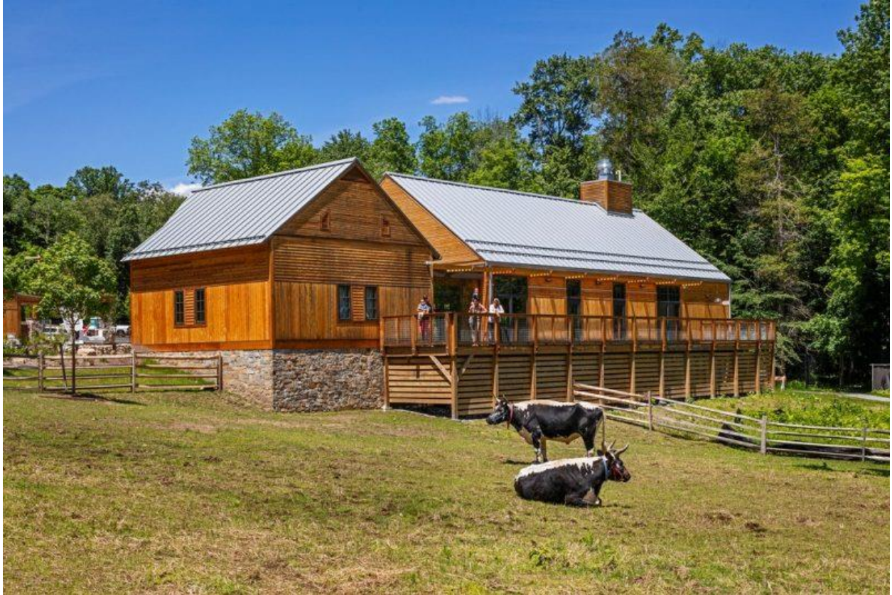
Farmhouse Education Center - Stamford Museum and Nature Center / TSKP Studio Photographer: Richard Barnes Photography
