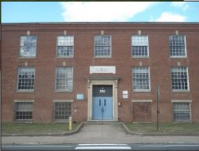
Before and After - Historic Cheney Building
