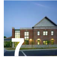
The Lexington School Lower School Wing Lexington, KY Photo Credit: Woodruff / Brown Photography
