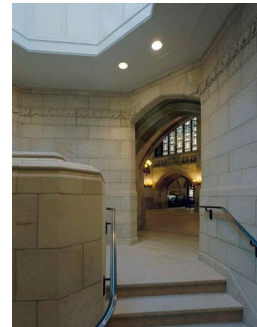
Newly inserted stairs connecting Bass and Sterling libraries, left.
