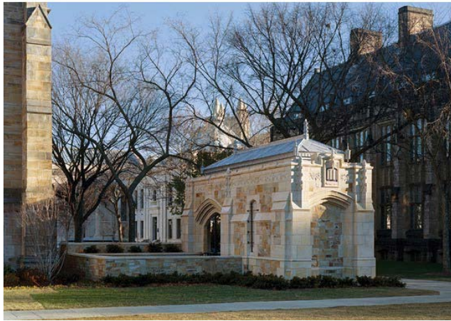
New accessible entry pavilion, above, and stair to below grade main entrance, right, designed to fit seamlessly with the architecture of James Gamble Rogers.
