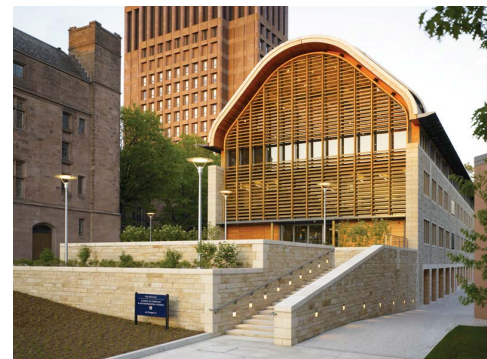
West Elevation facing Prospect Street, across from Ingalls Rink. Philip Johnson's Kline Biology Tower is in the background and Sage Hall is adjacent.
