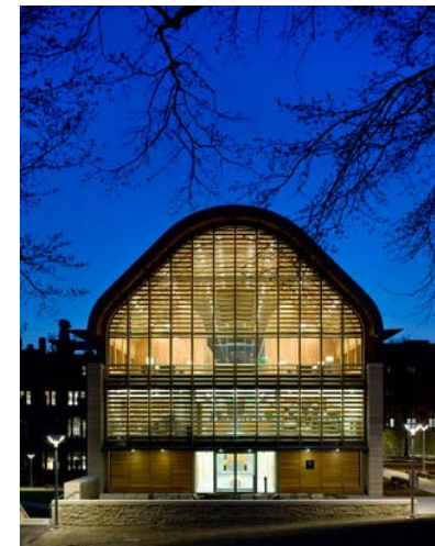
East Elevation facing Science Hill, at night. The building site had no "rear" entrance and an underground service node was built to service Kroon and the adjacent buildings.
