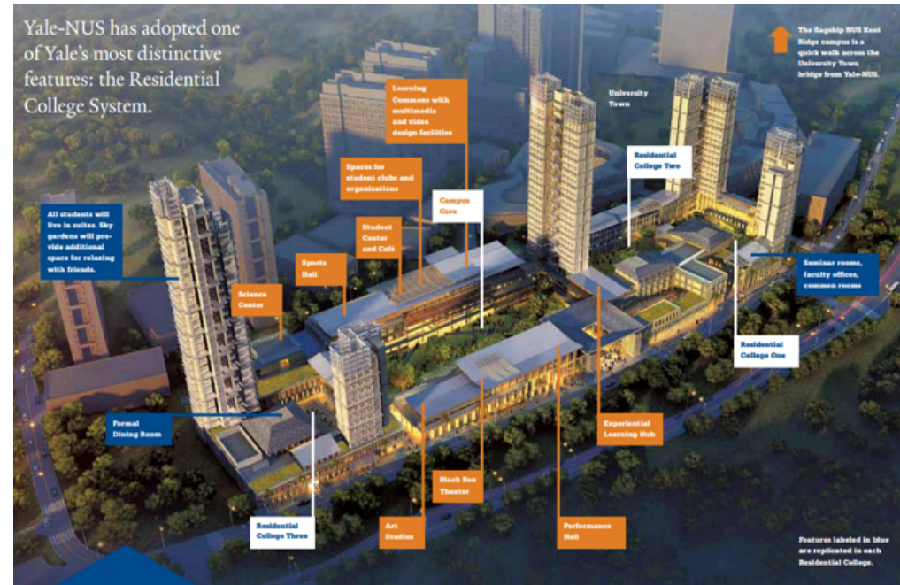
Yale-NUS College in design, above, and in construction, below.
