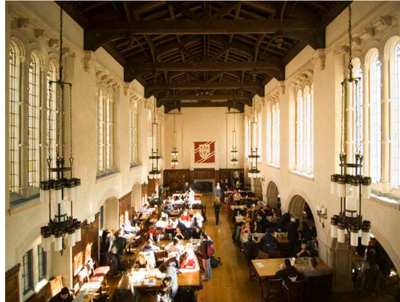
Restored Dining Hall with new acoustic plaster. Historic lighting fixtures were updated with new lamps, the lead camed windows and woodwork were restored.
