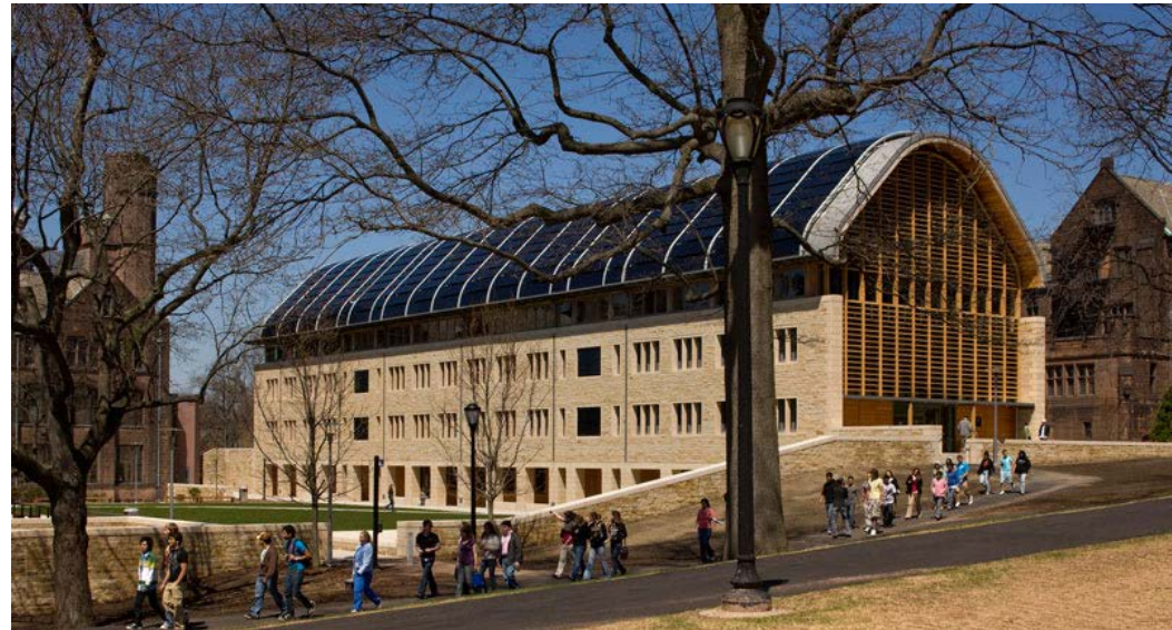
South Elevation, with students walking on Science Hill, location of Kroon's geo-thermal wells, the first at Yale
