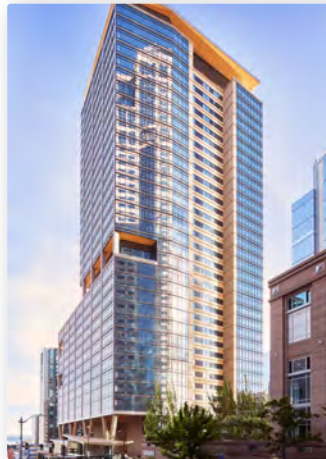
The building is structured around a side core, expressed on the eastern side of the tower, above the main lobby entrance
